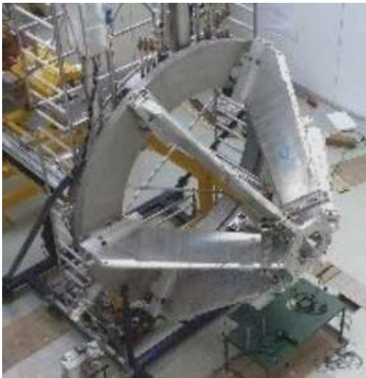
Figure 2.4: The superconducting magnet of HADES during its installation phase. The coils of the magnet are mounted on two support circles leaving space for RICH detector and free path for the beam axis in its center of symmetry as well as for tracks of particles produced in case of interaction. No detectors were installed at the time when the photograph was taken.
